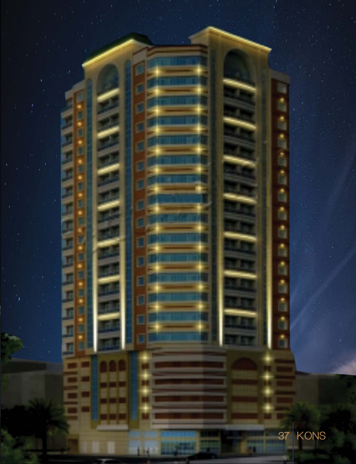
Building 15 - Floor, Ajman
